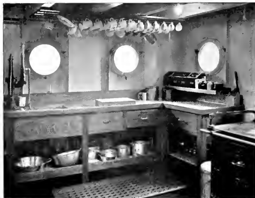
The electric galley of the new diesel-electric tanker J. H. Senior.
